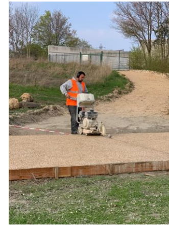
Sciage des joints
