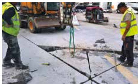
Excavation partielle
