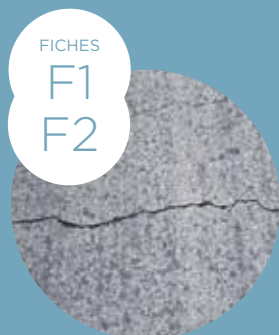
FISSURE TRANSVERSALE
