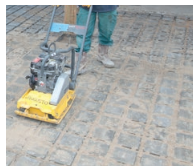
Photo 83 - Damage des joints.
